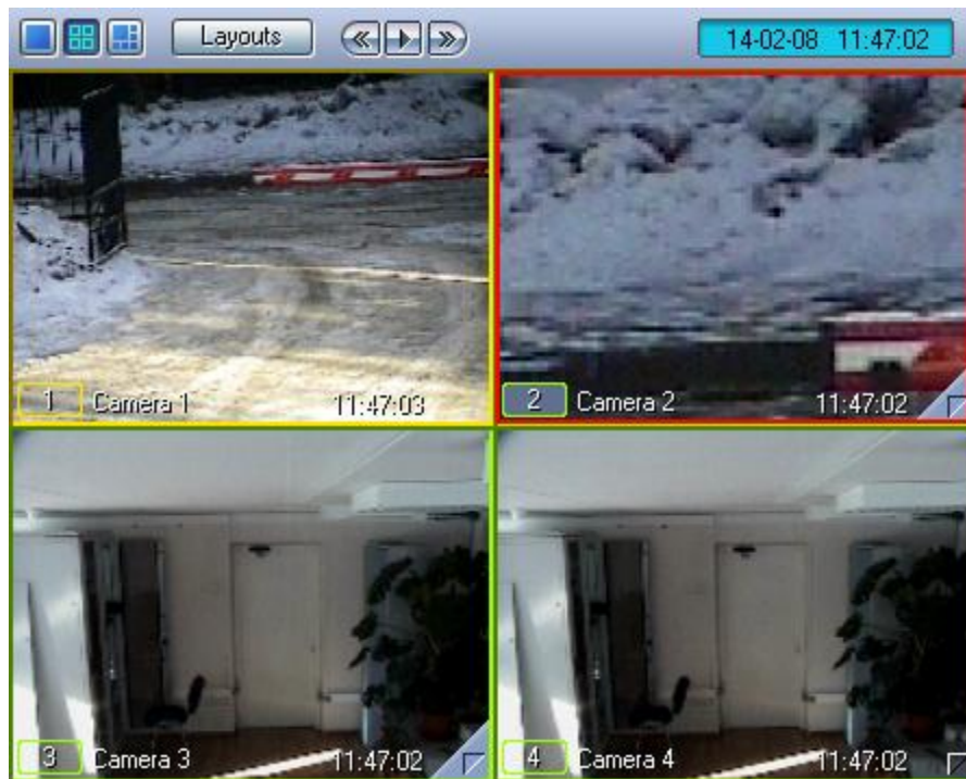
Fig. 4.3-7 Image dragging in the surveillance window
